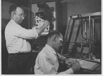
FORCE OUTPUT characteristics of small explosive devices are measured by Arnold Strasburg (left) and Oscar Braune (both 5524-2) who use a ballistic pendulum which they designed to evaluate rates of deterioration. The device is extremely accurate.
